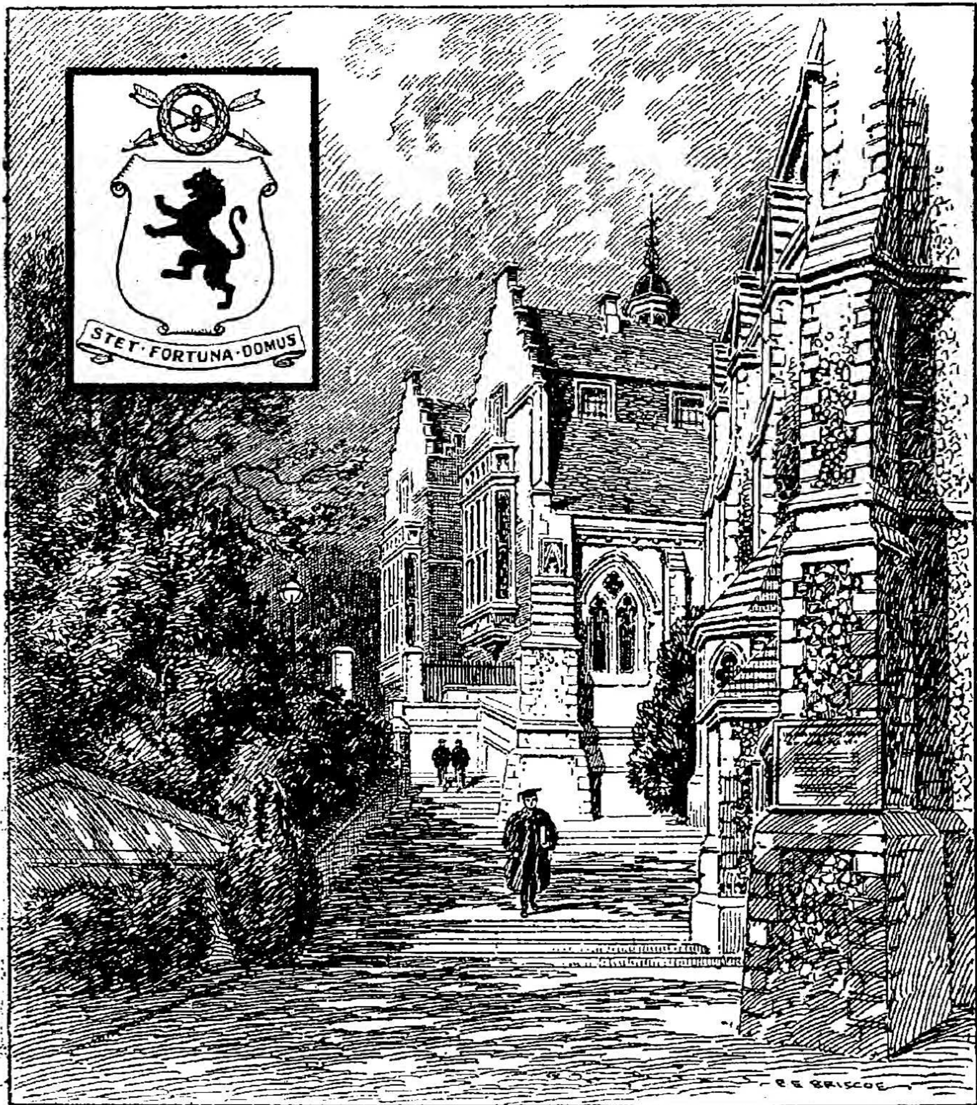
THE OLD SCHOOL AND CHAPEL, FROM THE TERRACE.
